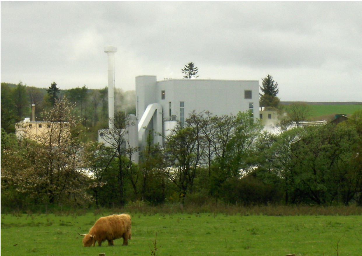
(Helius CoRDe biomass fired plant in Rothes, Morayshire – Scotland).
